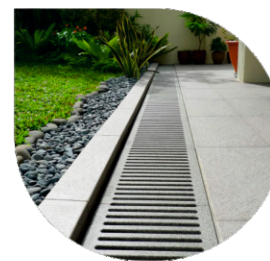
Rcc Steel Concrete Drainage
