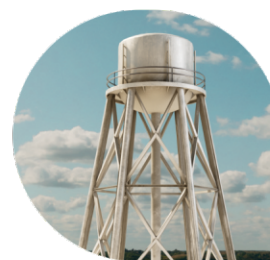
Over Head Water Tank
